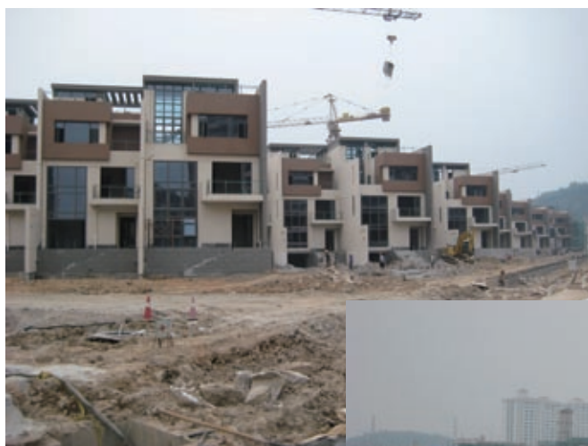
Town Houses of Yayao Oasis Phase 1, - construction works in progress
