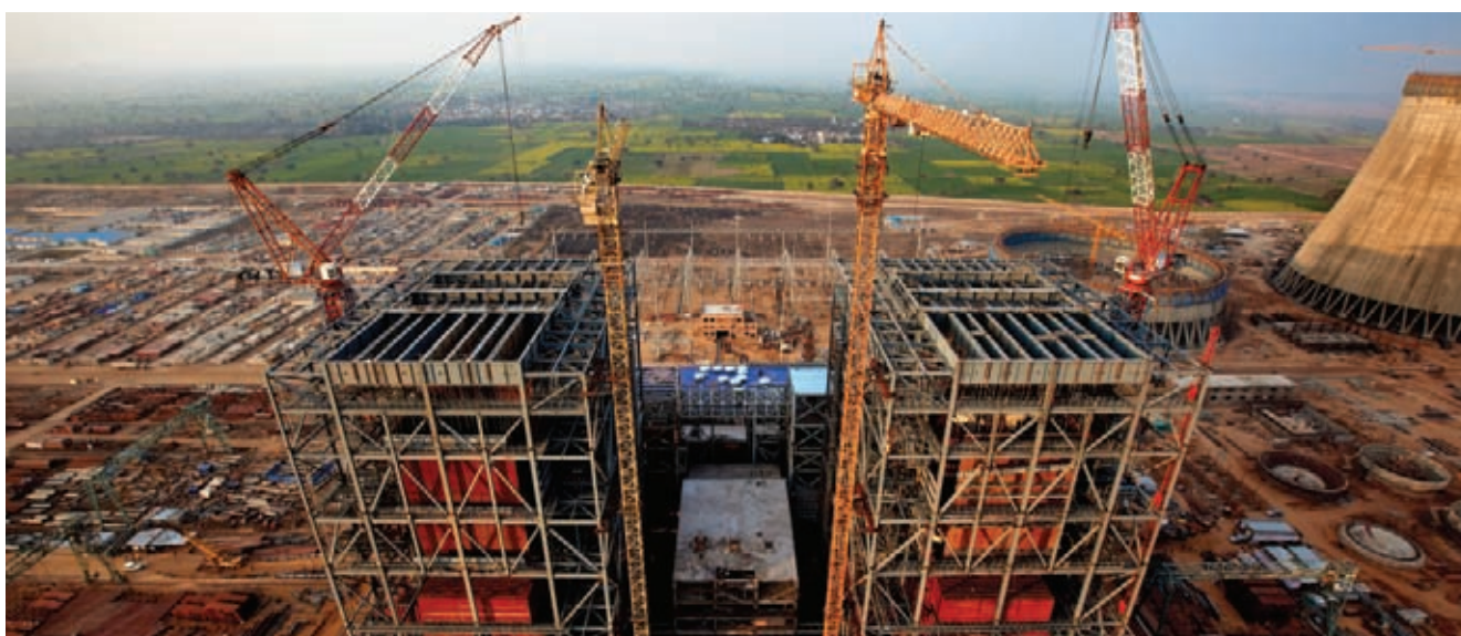
The Jhajjar Project under construction
