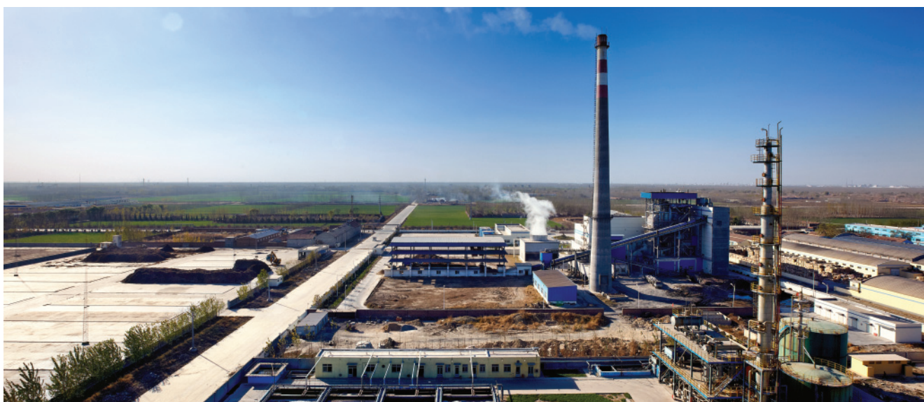
Shandong Boxing Biomass Plant
