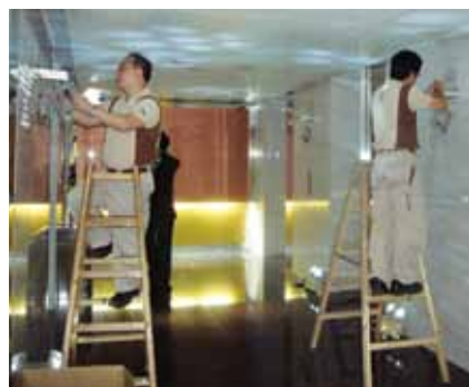
Installation of LED lights at 248 Queen's Road East
