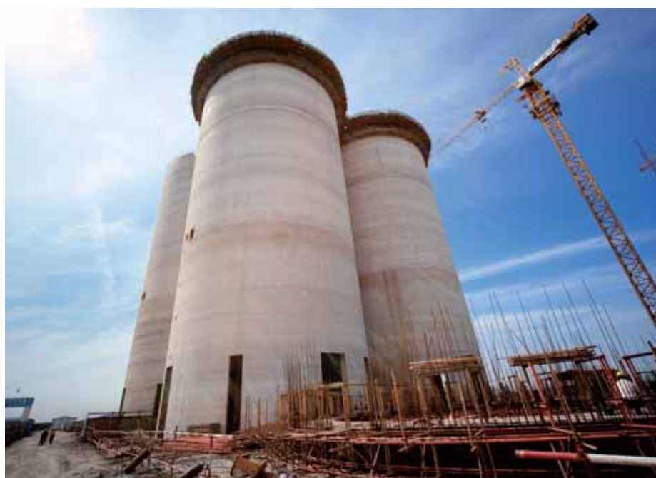
► Newly built silos at COFCO Excel Joy (Tianjin) Co., Ltd.
