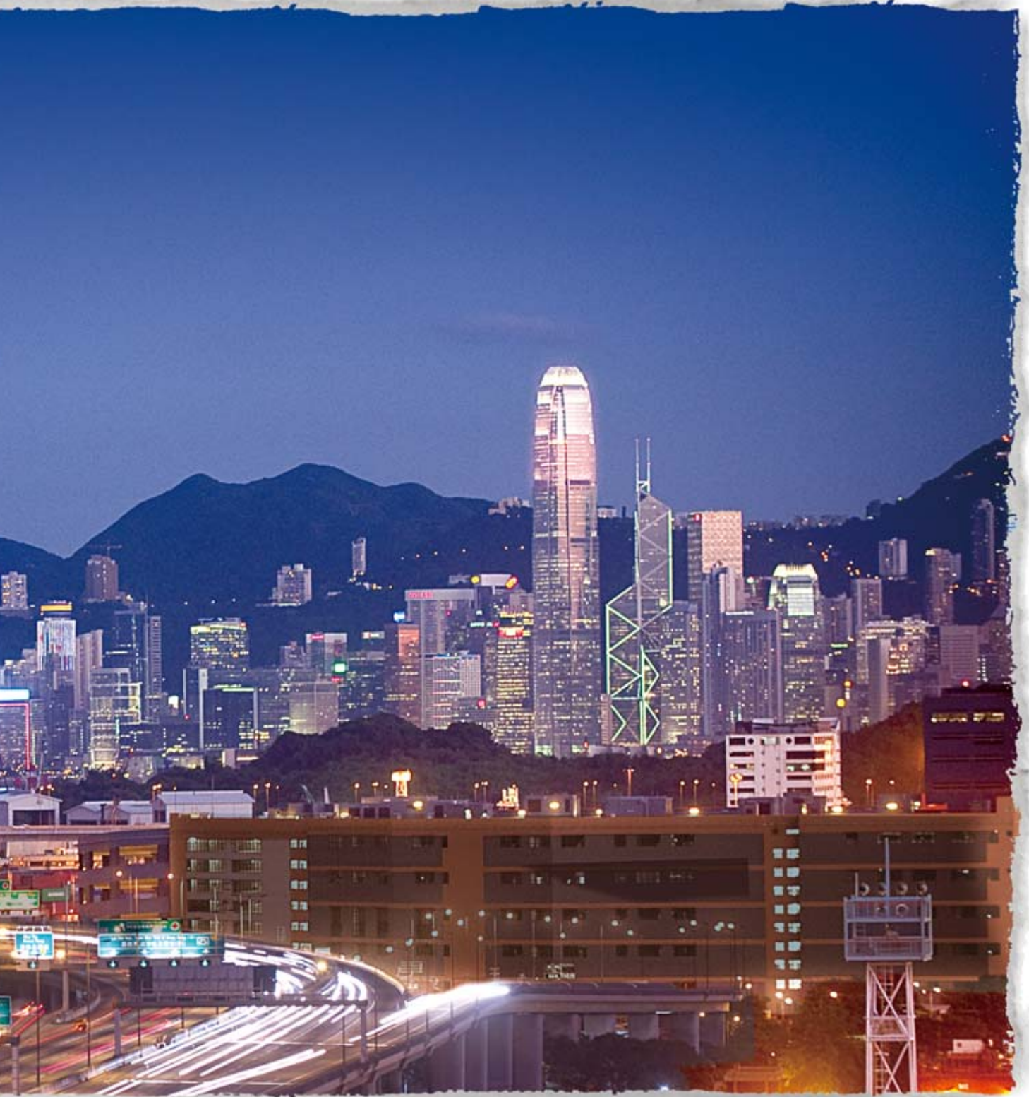
International Commerce Centre, Kowloon Station (left) and International Finance Centre, Central (right)
