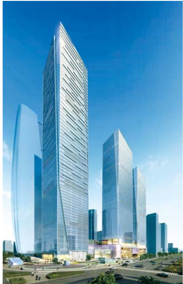
Nanjing ICC in the commercial core will include offices, a hotel and a shopping mall
