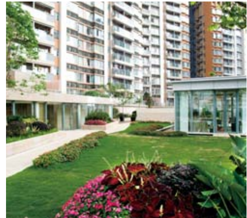
Green elements at The Latitude in southeast Kowloon provide a comfortable environment
