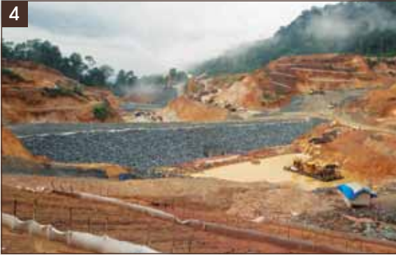
Tailings storage facility – 1st stage lift
