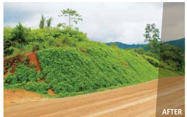
Roadside area rehabilitation (before and after).
