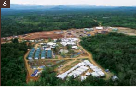
Camp and infrastructure area
