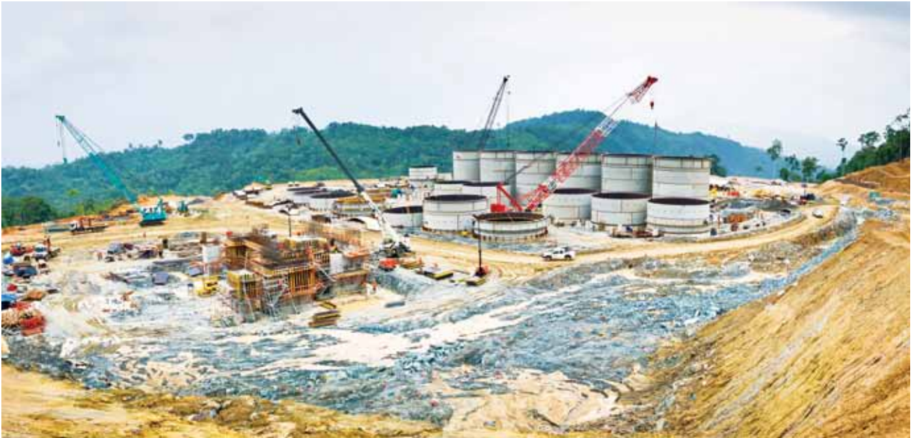
Plant site under construction.
