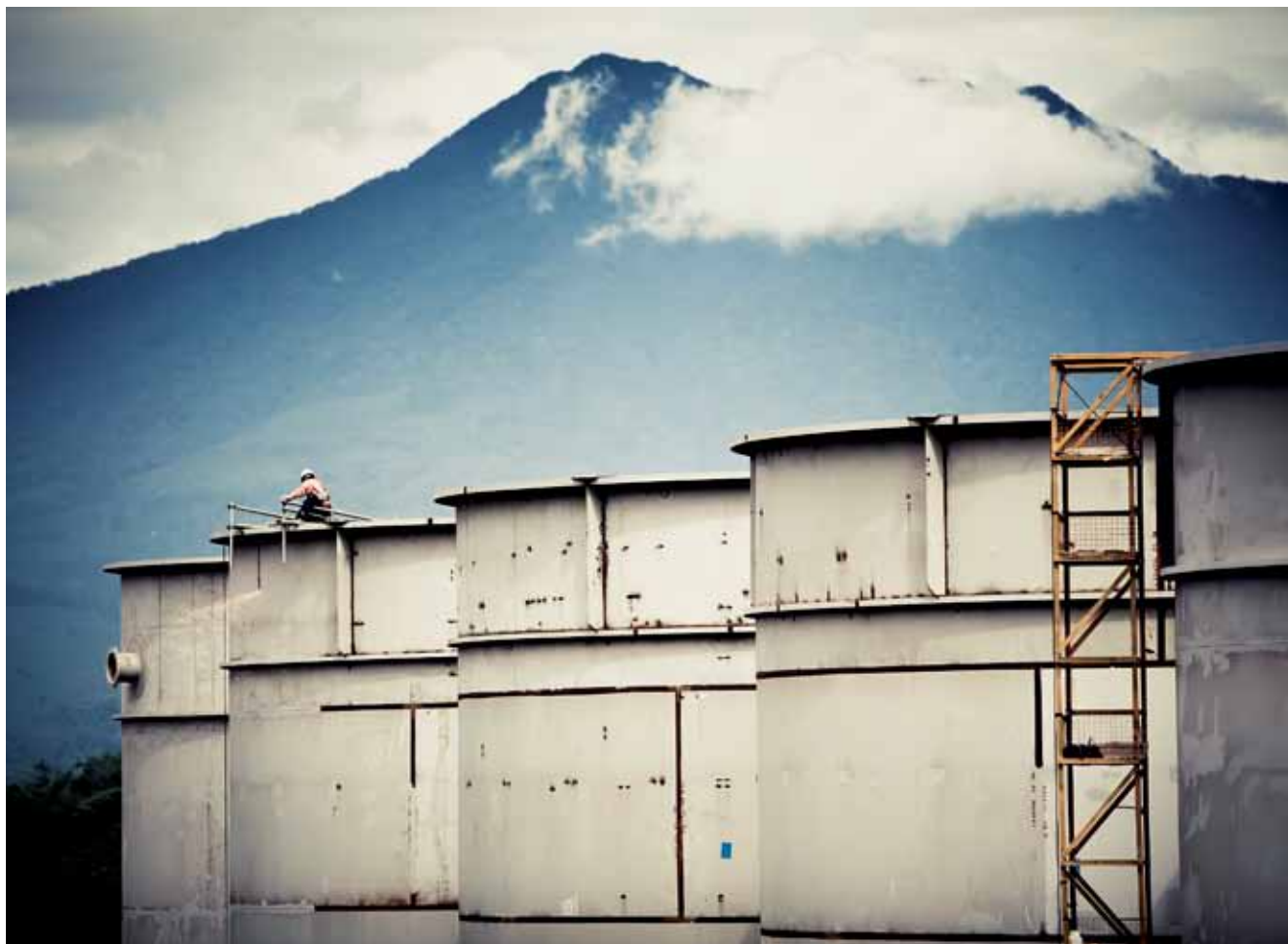
CIL tank erection.
