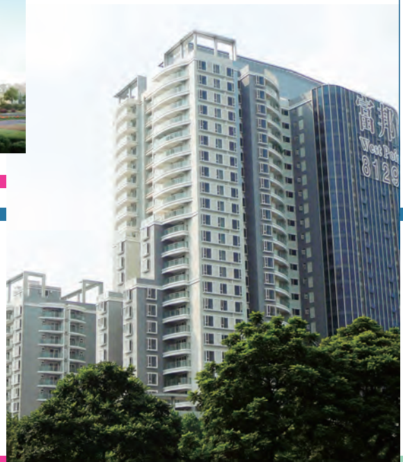
Guangzhou West Point Centre
