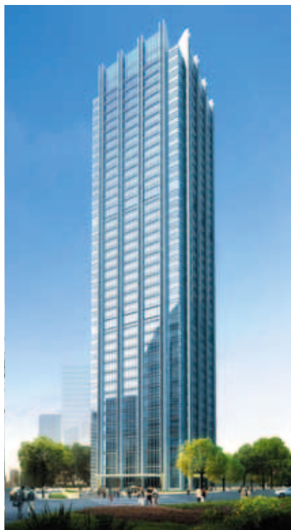
▲ Guangzhou Eastern Place Phase V - Office Block
