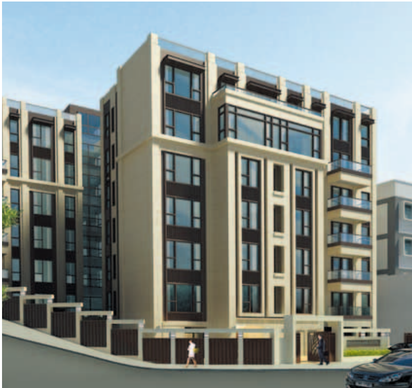
▲ Tai Hang Road Project
