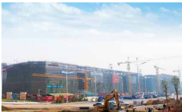
Construction at CSC Nanchang in full-swing 南昌華南城建設如火如荼
