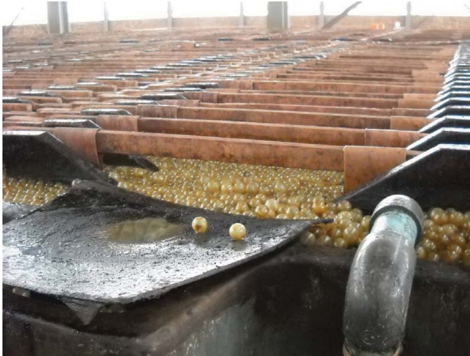
Figure 64: Electro Winning Cells in the Tank House
