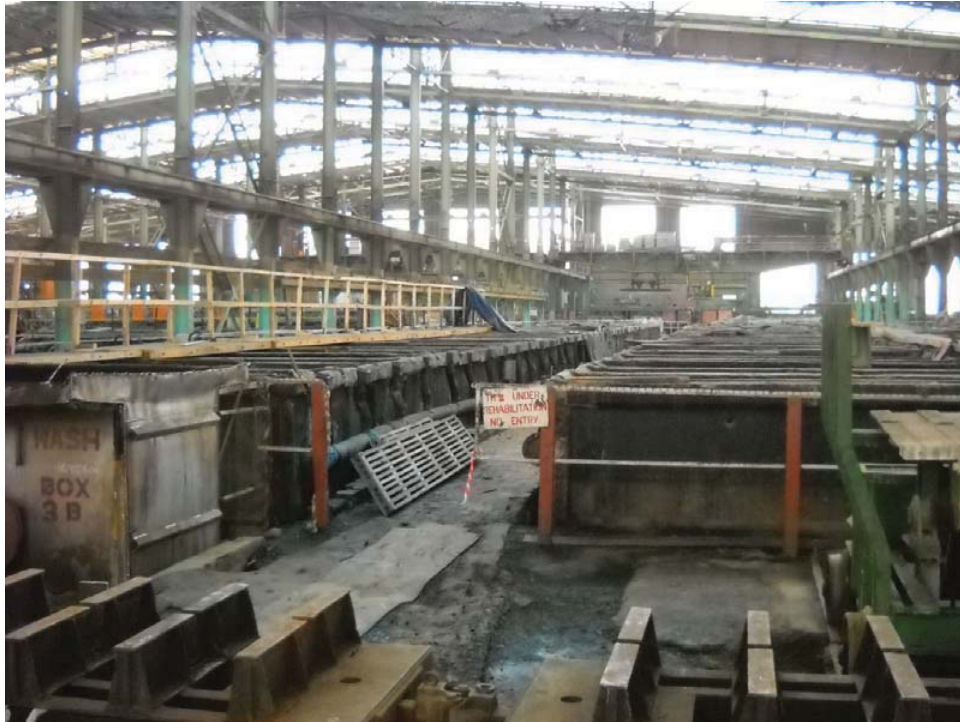
Figure 61: The Closed Module 2 of the Tank House
