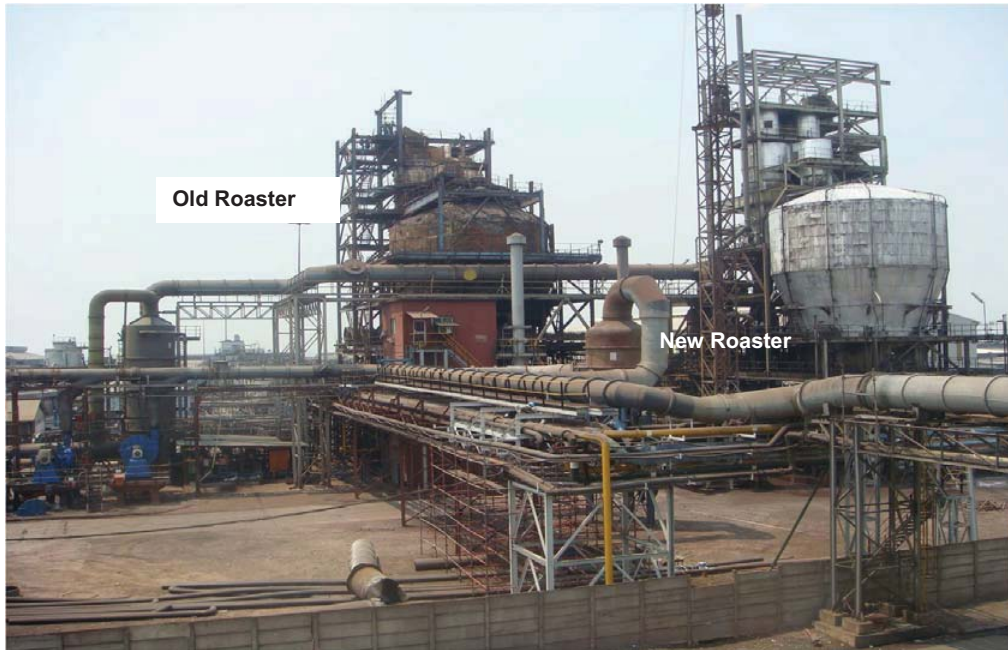
Figure 40: Old and New Roaster at Nkana Cobalt Plant
