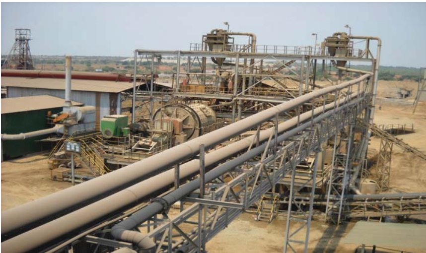
Figure 42: "Oxide" Plant Mill Installation
