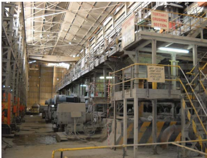
Figure 49: Secondary and Tertiary Crusher Building
