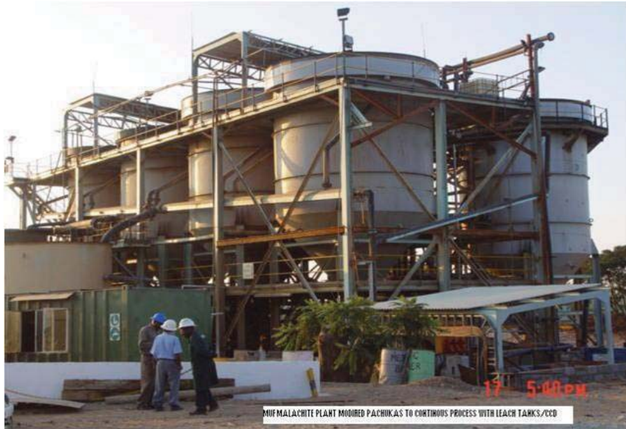
Figure 62: Leach Facility at Mufulira
