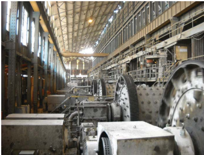
Figure 39: Mill Building at Nkana
