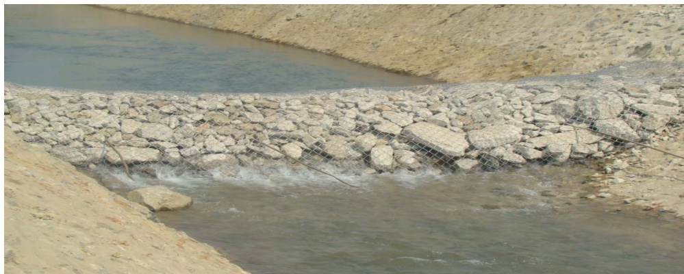
Figure 72: Solids settling ponds for wastewater leaving plant area
