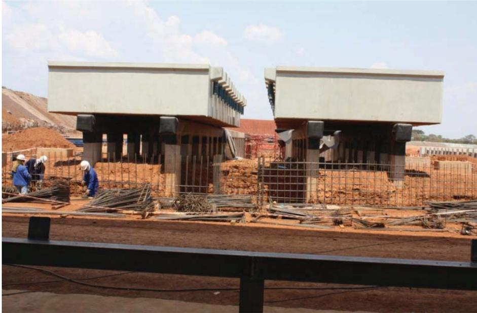
Figure 64: 40 000 tpa Module Electrowinning Cells Already in Position
