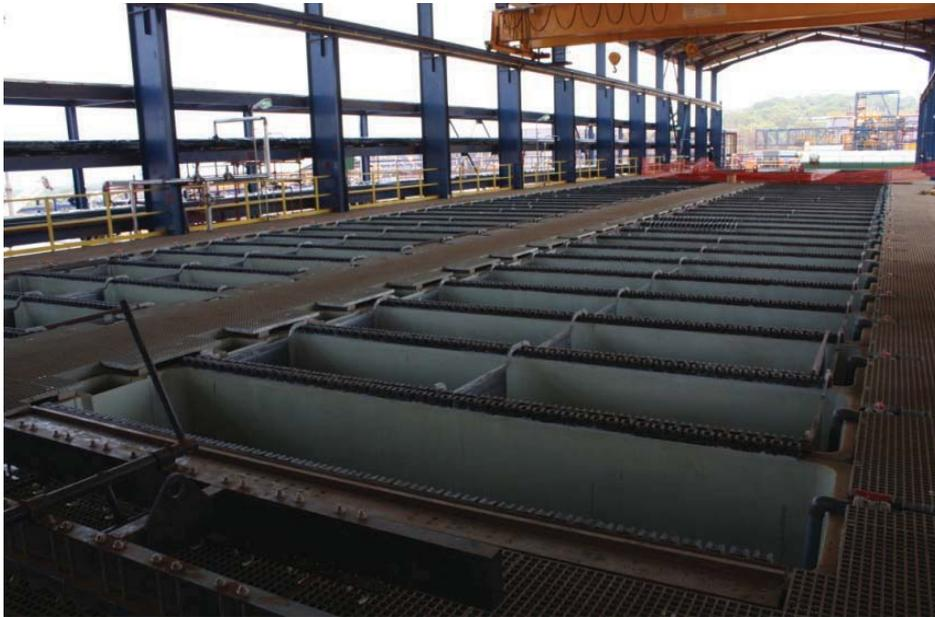
Figure 59: Tank House Inside during construction
