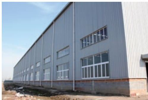
Steel processing plant in Tianjin
