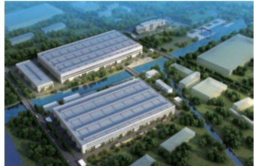
Bird-eye view of electrolytic tin plate manufacturing plant in Jiangsu
