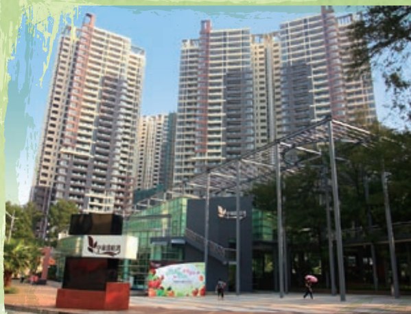
Guangzhou - Banyan Bay
