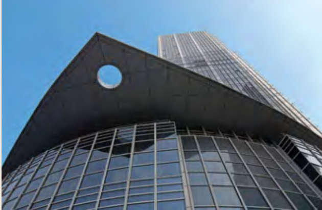
Chong Hing Finance Centre, Shanghai
