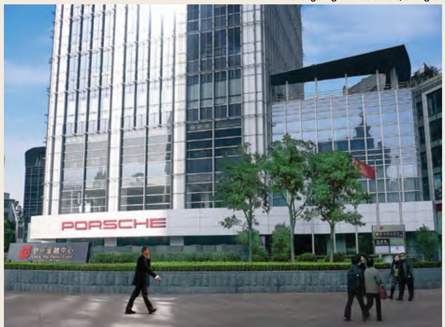
Chong Hing Finance Centre, Shanghai
