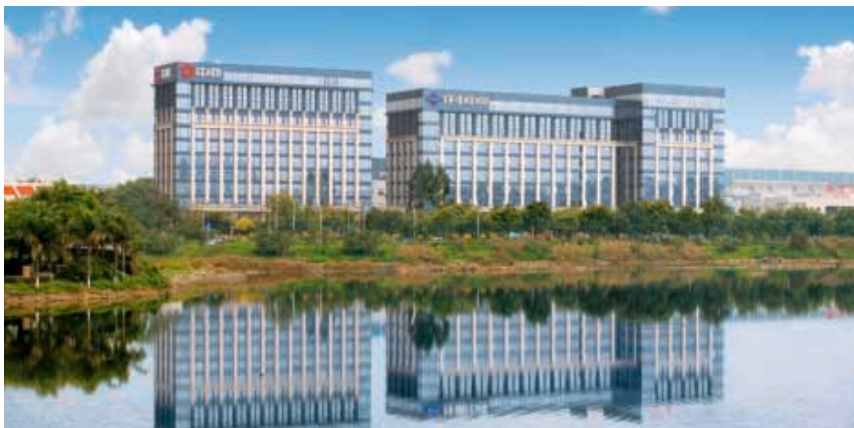
Xiamen • SCE Building
