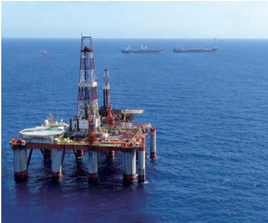
Wenchang platform with shuttle tankers in the distance, at Wenchang field in the South China Sea.
