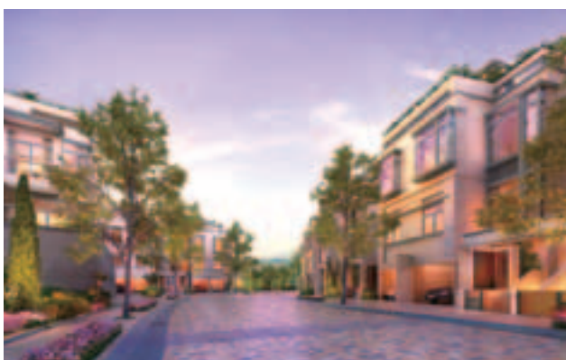
The Green, Fanling, Hong Kong
