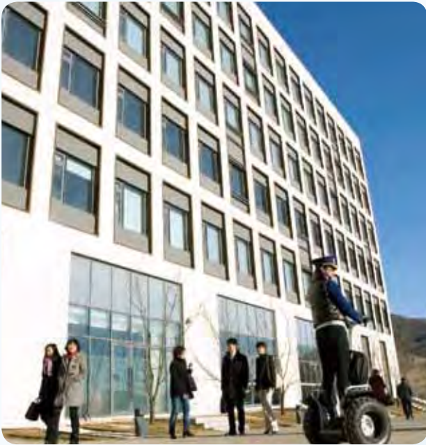
Software offices in Dalian Tiandi
