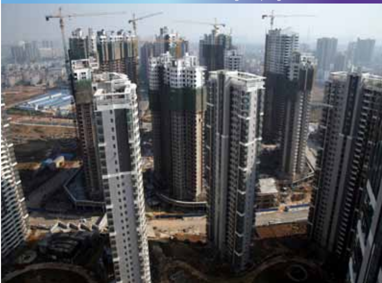
Residential buildings in progress in Beichen Delta
