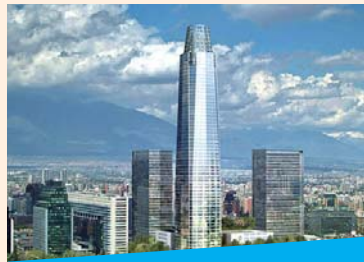
▲ Chile – 2G/3G Wireless Enhancement Project for Costanera Centre (the tallest building in South America)
