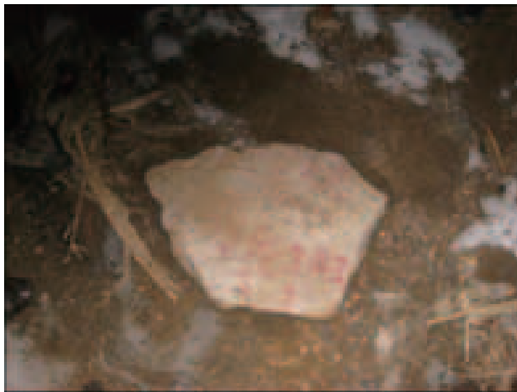
Figure 7-10: Concrete cap on collar of ZK1202
