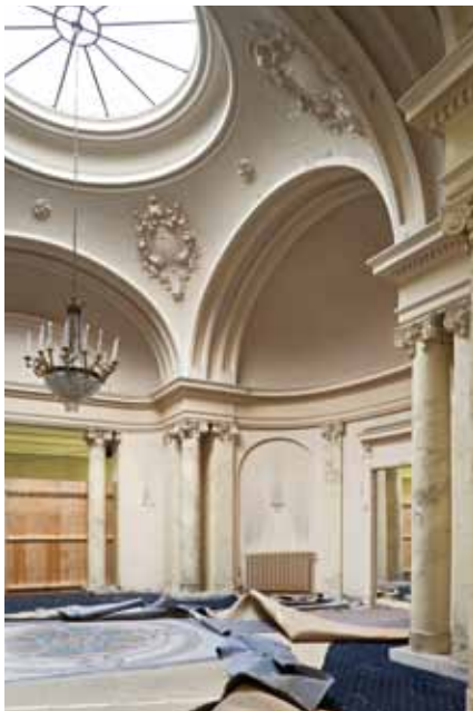
Above: Renovation in progress inside the building.
