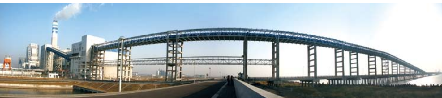
1000MW Thermal Power Station in Caojing
