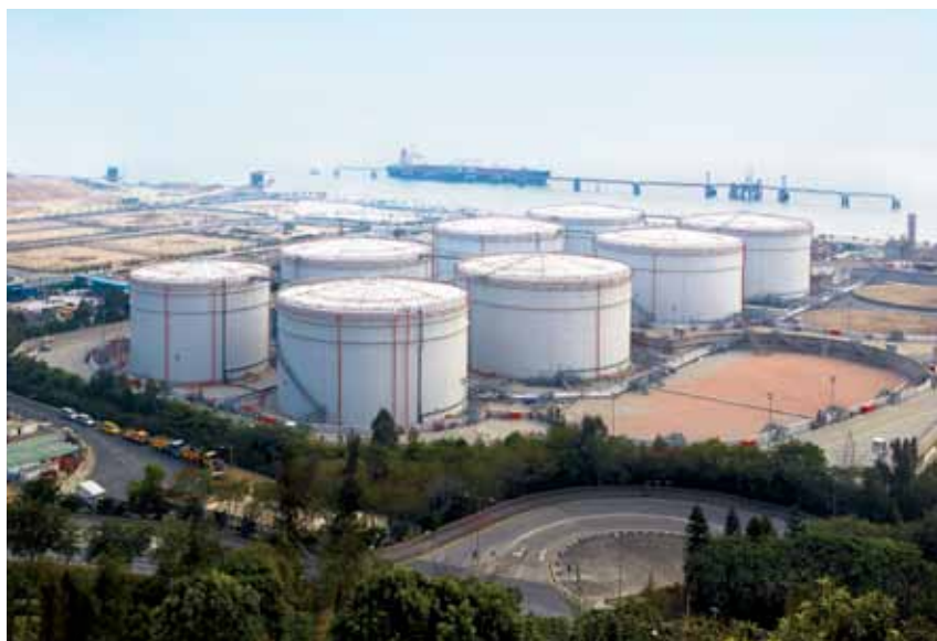
ECO Environmental Investments Limited (ECO)'s Aviation Fuel Facility in Tuen Mun
