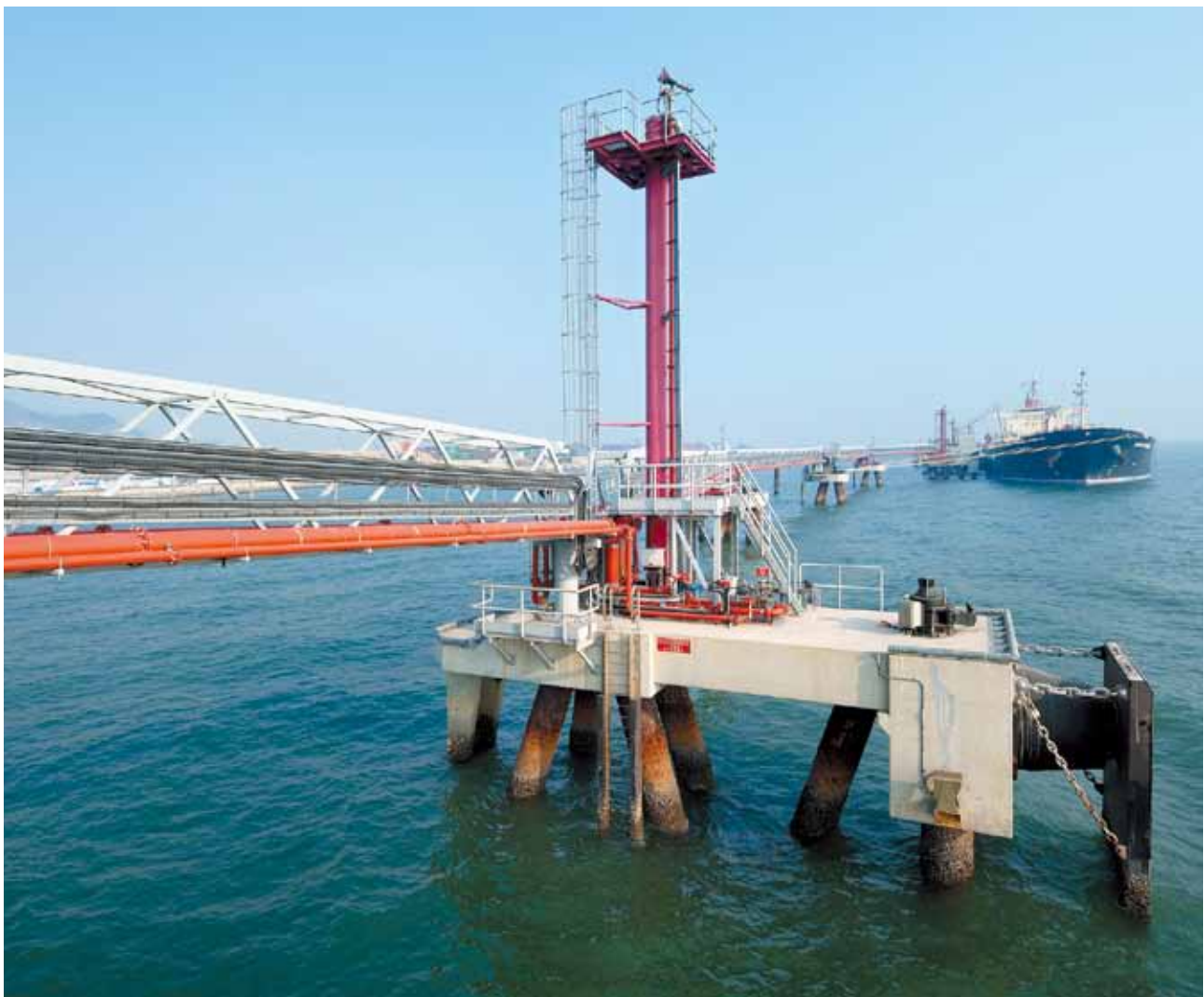
Eco Aviation Fuel Facility consists of two jetties for berthing tankers
