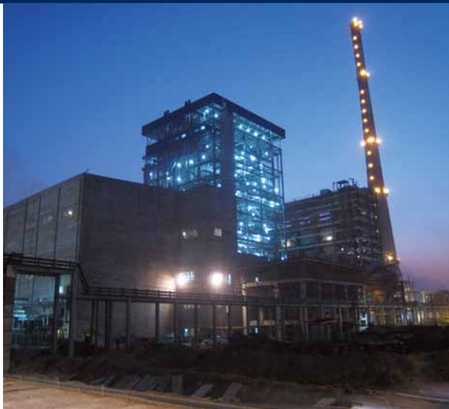
Indian Dugarpus Power Plant Project
