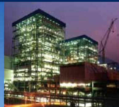
600MW Supercritical Boiler in Qinbei Power Plant, the first of its kind in the PRC
