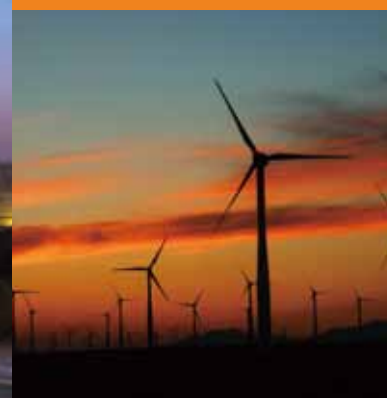
Arac Power Plant (4 x 325MW) in Iran
