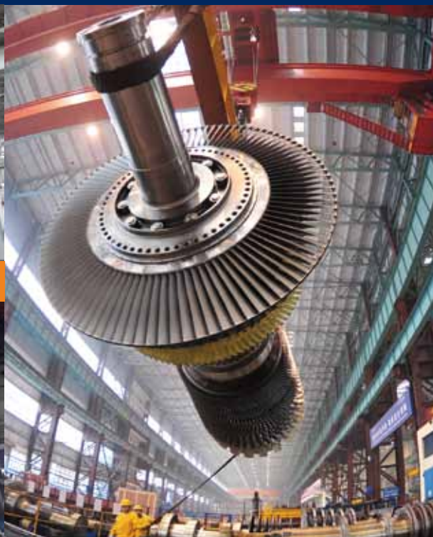
Hoisting of gas turbine rotor
