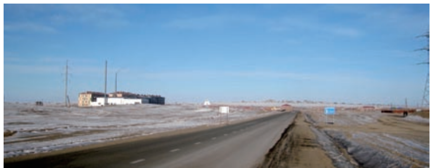
Paved road from Tavantolgoi airport to the miners' camp
