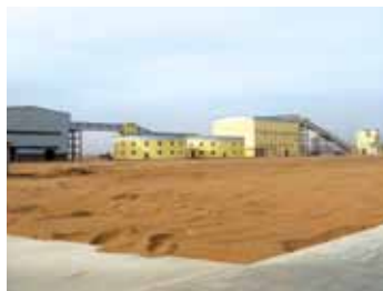
Wet wash plant at Ceke
