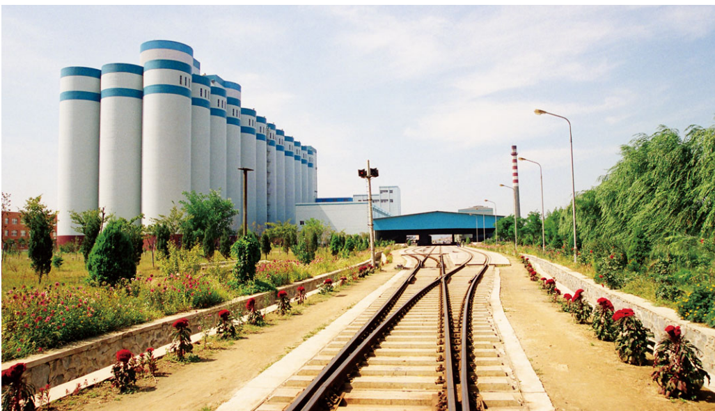
► Dedicated railway for brewing materials at COFCO (Dalian) in Liaoning
