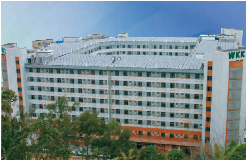
Worker dormitory, Dongguan 工人宿舍，東莞
