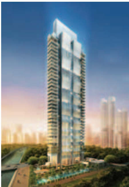
Perspective of Centennia Suites, a property development project in Singapore
