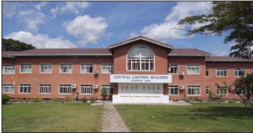
Figure 12-3: NFCA Office Building ("Central Control Building")
