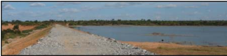
Figure 8-4: An Overview of the Chambishi TSF
