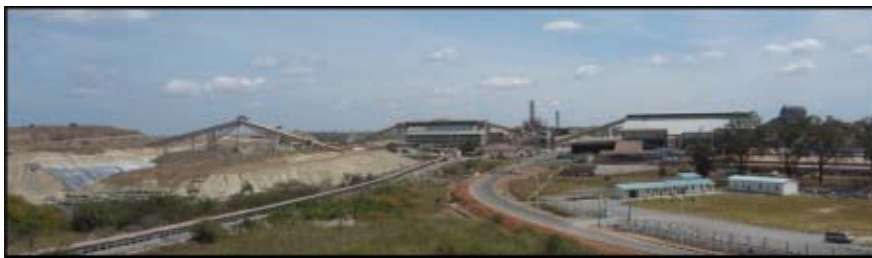
Figure 8-1: An Overview of Chambishi Processing Plant
