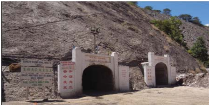
Figure 7-3: Portals of Main Ramp of Chambishi West Mine
