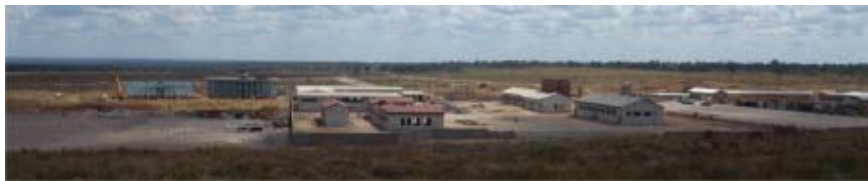
Figure 8-14: An Overview of Muliashi Leach Plant
