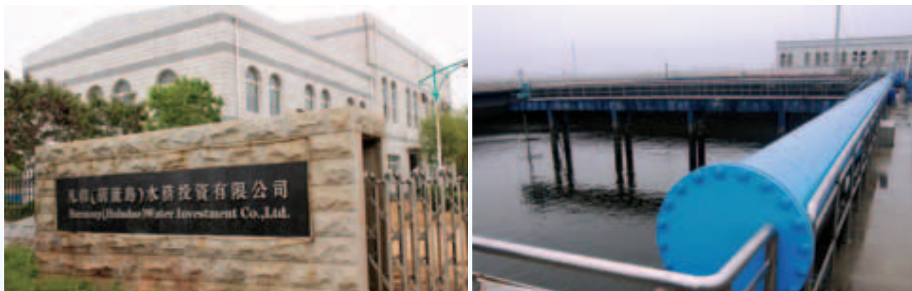
Our wastewater treatment plant in Hulu Island City, Liaoning Province, the PRC.
