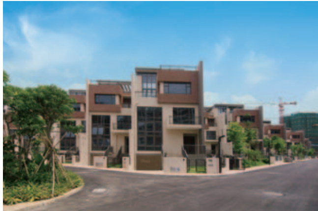
Partial view of town houses under Phase 1 of Metropolitan Oasis, Da Li District, Nanhai
