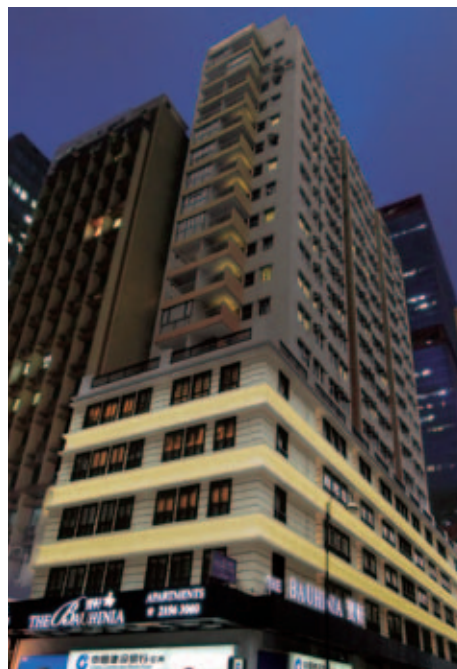
The Bauhinia Hotel (Central) and the serviced apartments upstairs
