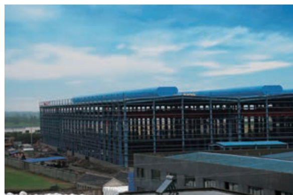
* ETP manufacturing plant under construction
