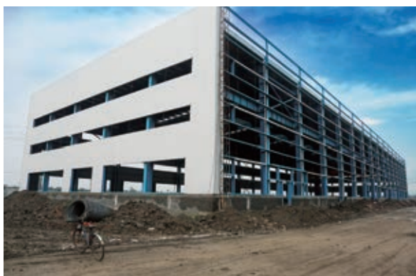
* Rolling mill workshop under construction (part of the ETP manufacturing plant)
