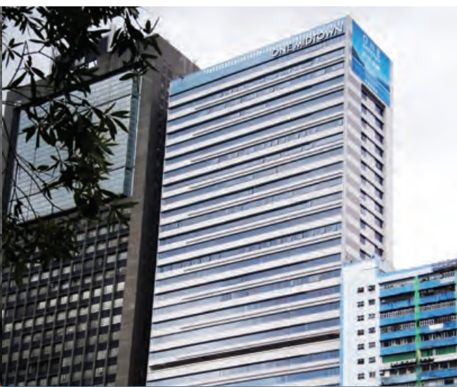
Proposed industrial development at TWTL No. 36 Hoi Shing Road, Tsuen Wan, New Territories – Design, supply and installation of aluminium window, window wall, canopy and aluminium cladding 新界荃灣海盛路TWTL36號的建議工業發展項目－設計、供應及安裝鋁窗、幕牆、簷蓬及鋁飾板
