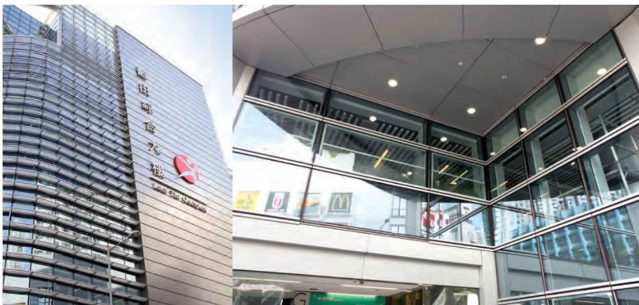
Lam Tin North Municipal Services Building – Design, supply and installation of aluminium curtain wall, aluminium cladding, canopy, skylight and feature 藍田北市政大樓－設計、供應及安裝鋁幕牆、鋁飾板、簷蓬、天窗及裝飾
