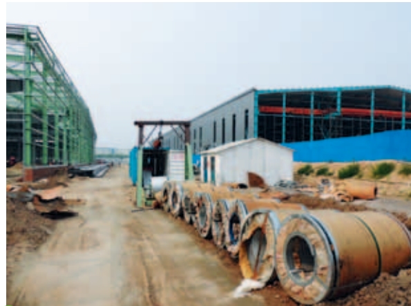
Taiyuan Processing Centre (under construction)
