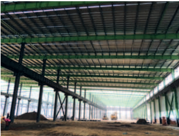
Taiyuan Processing Centre (under construction)
