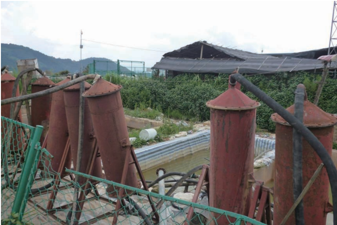
Adsorption, Desorption and Recovery (ADR) Plant
