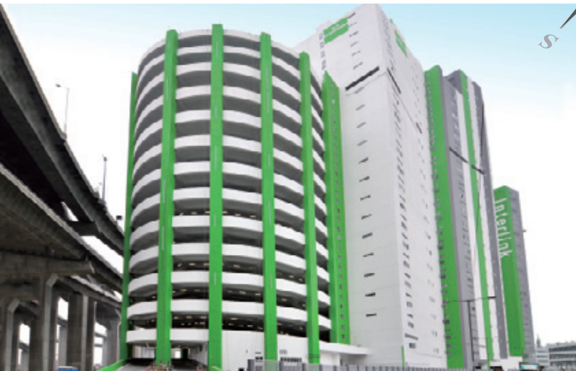
Interlink, Tsing Yi, a project undertaken by Hip Hing
