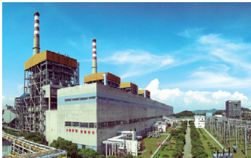
Zhujiang Power Plants
