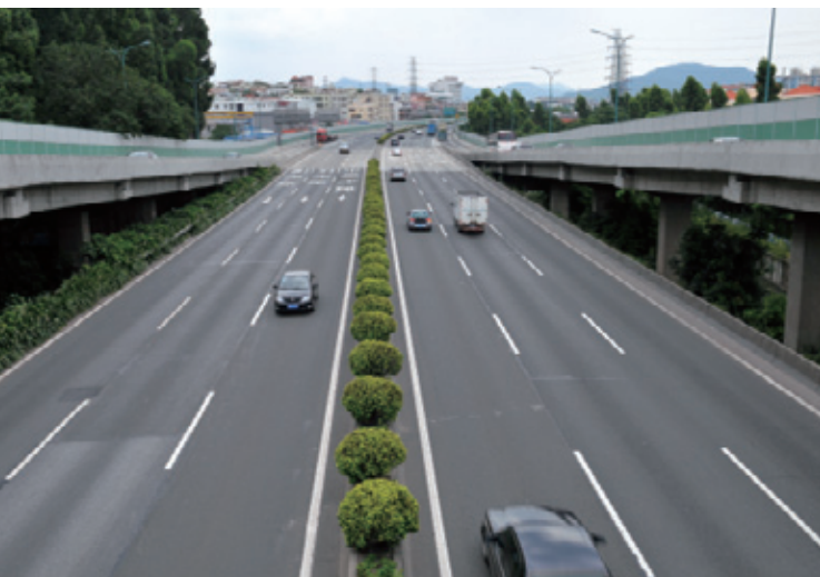
Guangzhou City Northern Ring Road
