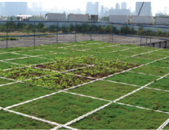
A green roof at a construction site office of Hip Hing.
