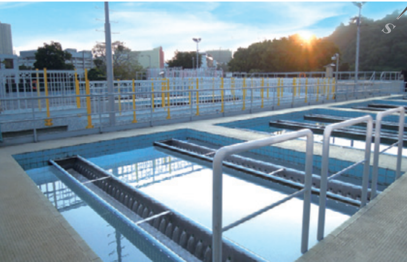
Macau Water Plant
