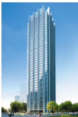
◆ Guangzhou Eastern Place Phase V - Office Block
