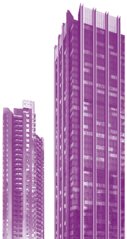
Cover Photo: Guangzhou Eastern Place Phase V, the Group's residential / office / commercial property located at Guangzhou, China
