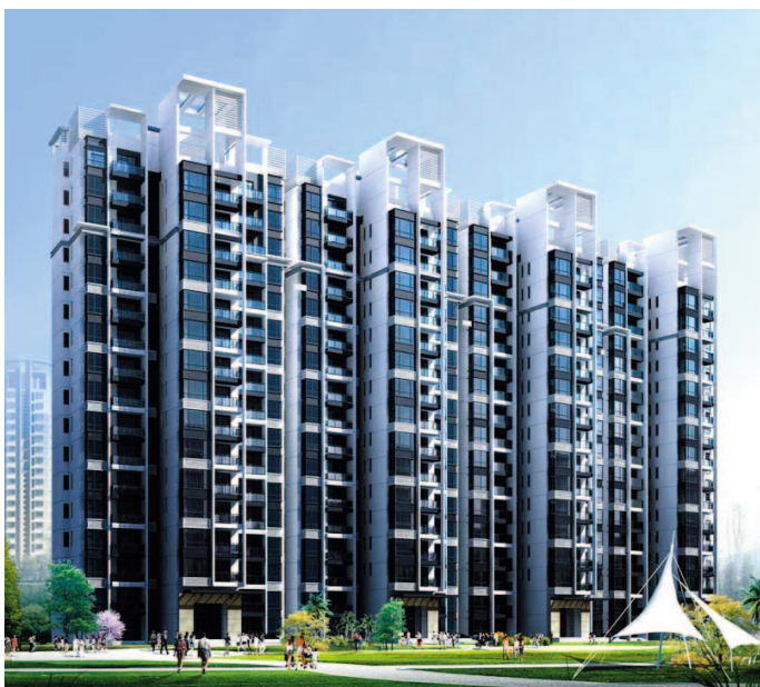
◆ Zhongshan Palm Spring — High-rise Residential Towers
