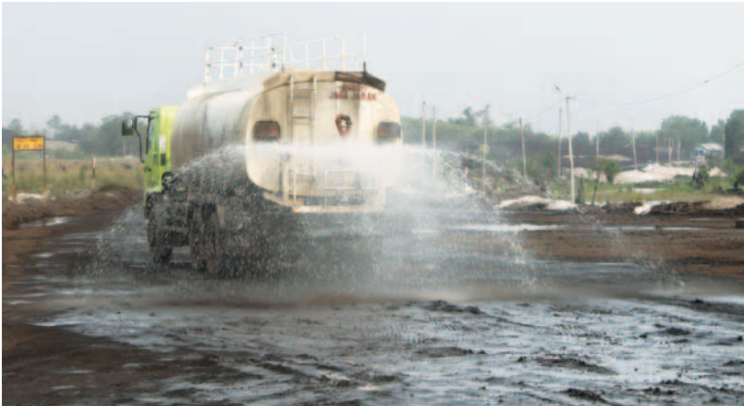
Upgrading and maintenance of coal hauling road
