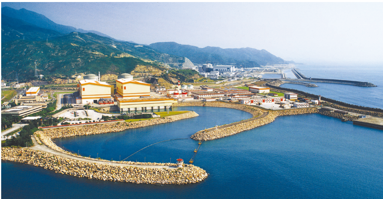
Supplying reliable clean energy to Hong Kong – Daya Bay Nuclear Power Station
