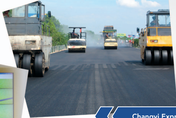
Changyi Expressway, Hunan
