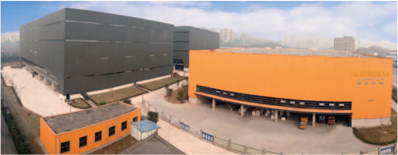
■ Phase 2 of logistics centre completed in Q4 2012, Chongqing, PRC
