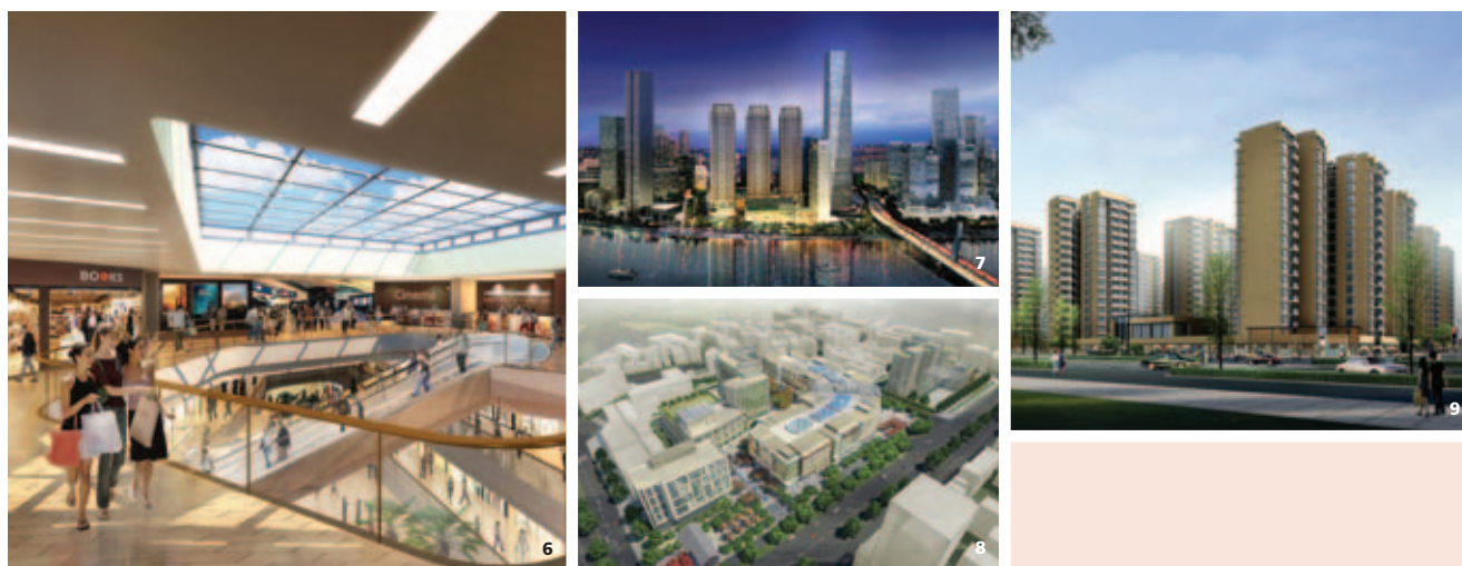
■6. Retail portion of Jing An Kerry Centre, Shanghai, PRC* ■7. Tianjin Kerry Centre, Tianjin, PRC* ■8. Hangzhou Kerry Centre, Hangzhou, PRC* ■9. Parkview Residence, Hangzhou, PRC*
