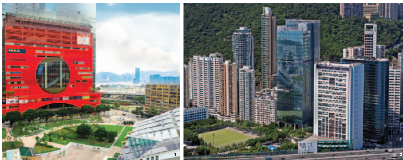
■ 1. MegaBox, Kowloon Bay, Hong Kong ■ 2. Kerry Centre, Quarry Bay, Hong Kong
