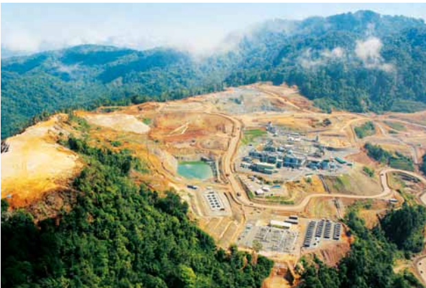
Aerial photo of Purnama on the left and the Process Plant.
