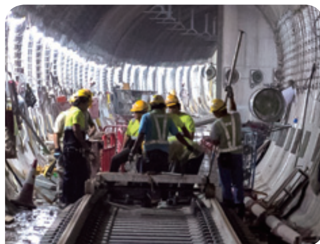
Track laying works commenced for the West Island Line
