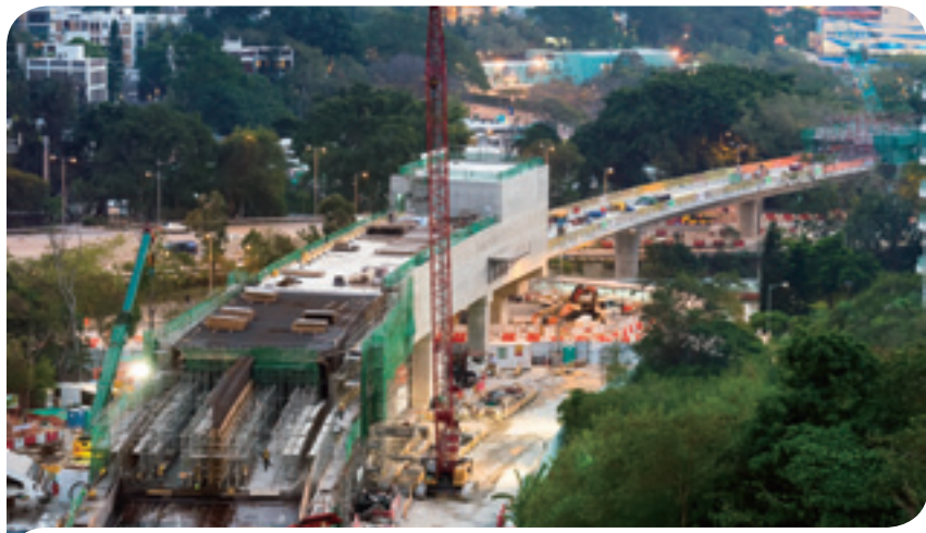
Construction of viaducts spans across southern district
