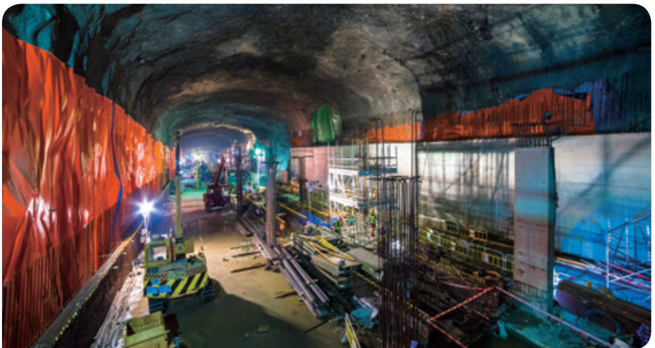
Tunnelling work forges ahead on the Hong Kong railway expansion
