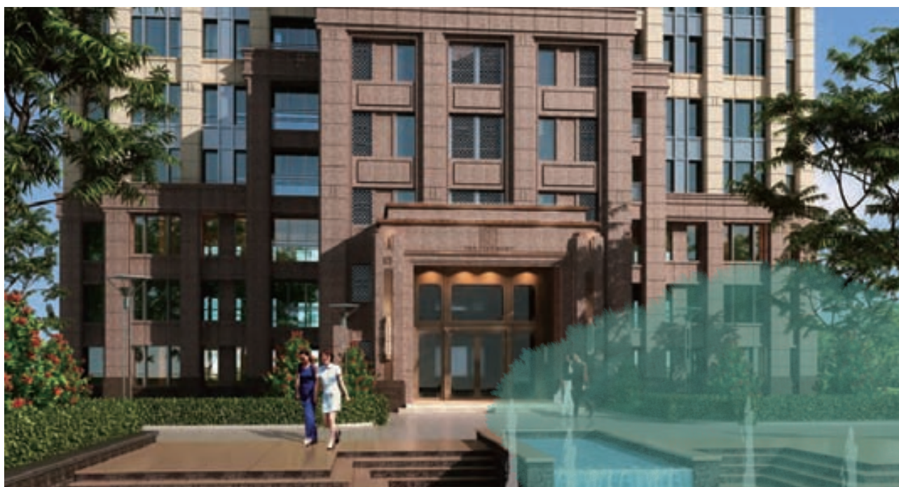
Garden view of The Piedmont, Guangzhou
