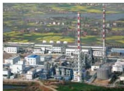
The production facilities in Hubei
