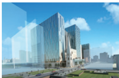
University of Montreal Hospital Centre, Montreal
