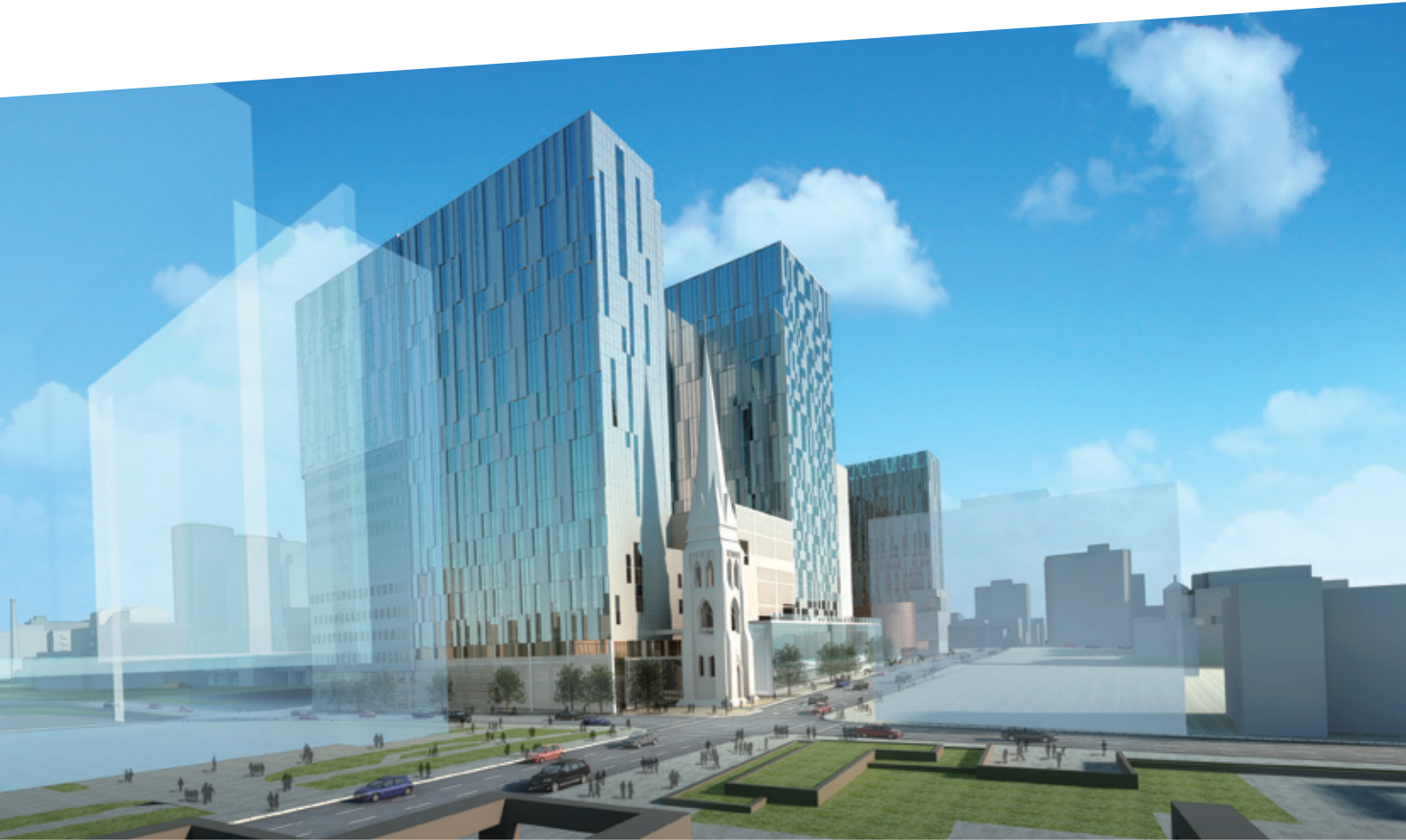
University of Montreal Hospital Centre, Montreal
